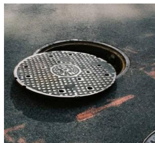
Fig 1: Newly mounted manhole at Trans-Amadi layout, Rivers State.
